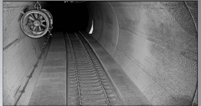
grey-scaled point cloud of subway tunnel
